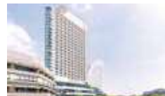
THE YOKOHAMA BAY HOTEL TOKYU
