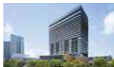
THE WESTIN YOKOHAMA
